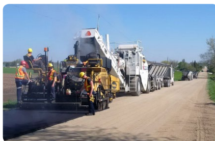
Streicher Line Paving Project in the Township of Wellesley.
