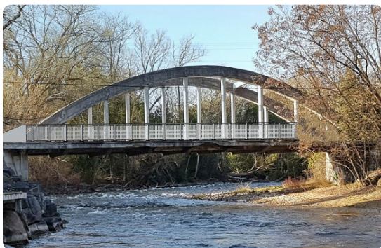
Rehabilitation of Black Bridge in the Town of the Blue Mountains.
