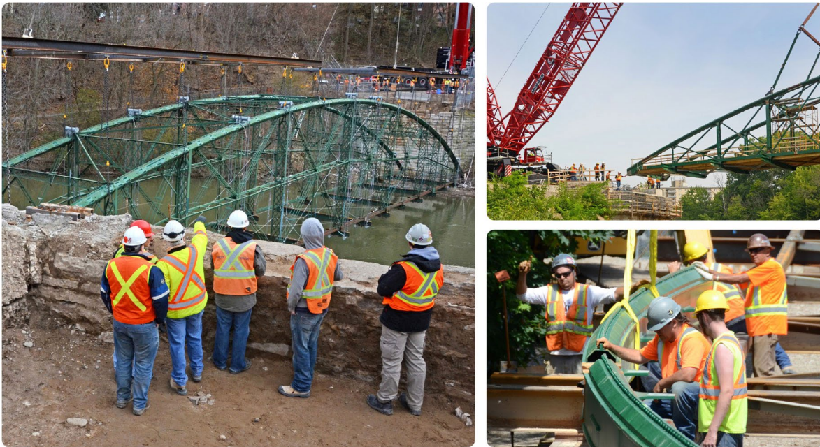
Rehabilitation of the Blackfriar Bridge in the City of London.
