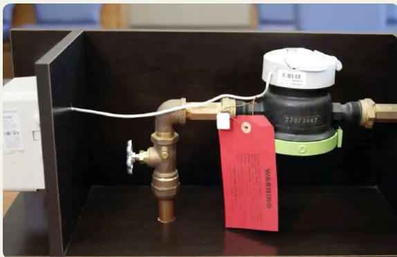
2018 Winner: The Town of LaSalle's Water Meter Replacement Project.
