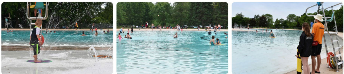
Kiwanis Park Pool Renovation in the City of Kitchener.
