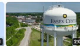
Essex's Harrow Streetscape Project
