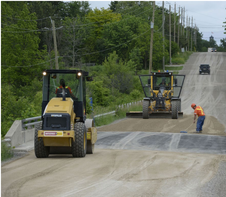
Township of Enniskillen, Tile Yard Road Reconstruction
