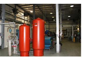
The Township of Terrace Bay invested in its water distribution system to help alleviate low pressure and ultimately reduce Boil Water Advisories for residents. The goal of the Pressure Vessel Project was to improve local water plant efficiency and realize energy savings.
